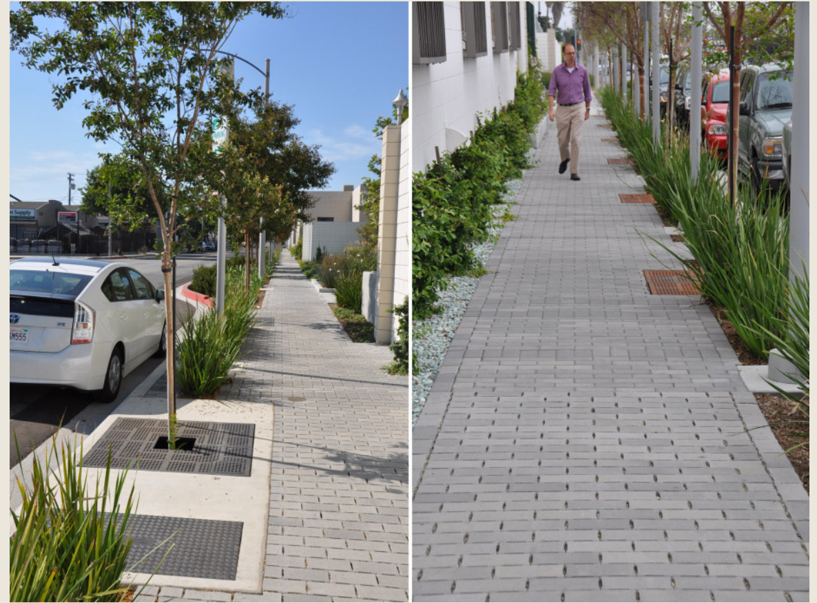
City of Burbank permeable sidewalks
