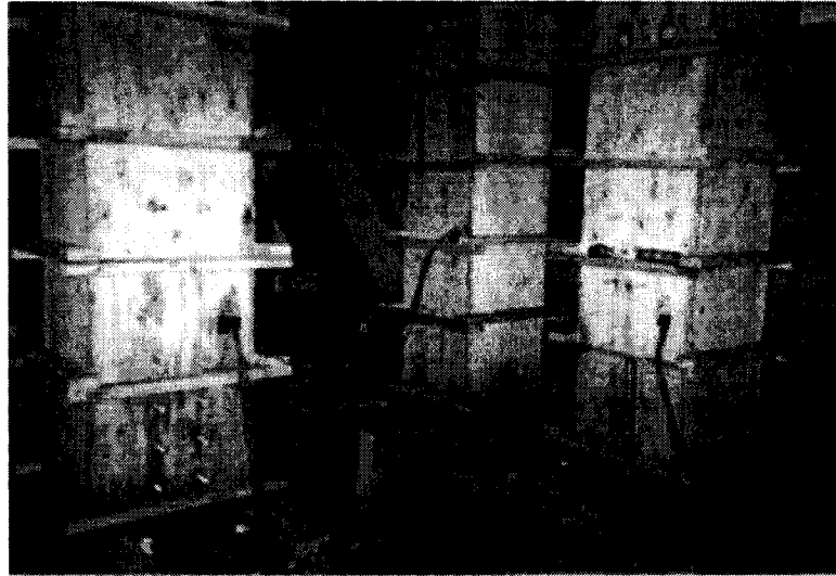
Fig. 3.12(b)-Formwork for columns (continued).
