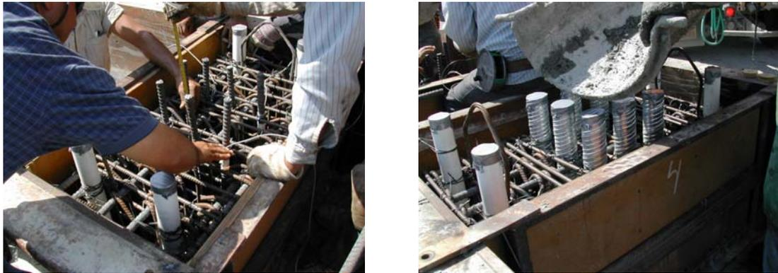
Figure 3.17: Steel cages of footings
