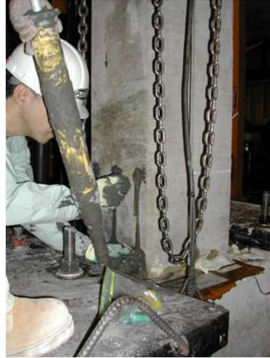
Figure 3.22: Filling of SS mortar into sleeves
