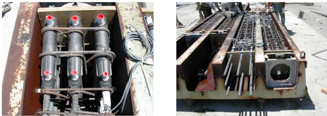
Figure 3.16: NMB splice sleeves and dowel rebars
