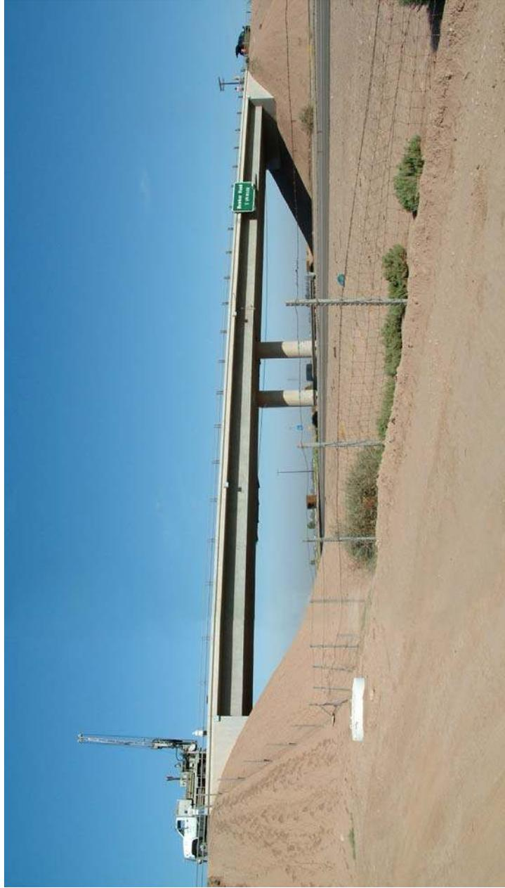
Figure 5.29: Tow-Columns Two-Spans Bridge
