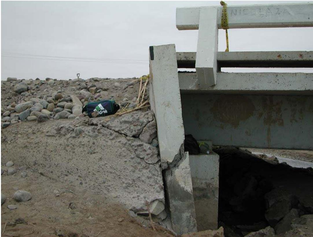
Figure 2.7: Backwall Shear Failure and Mobilized Passive Wedge
