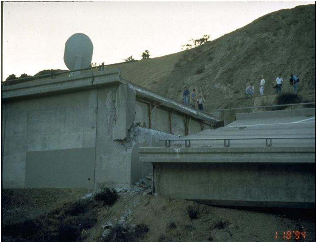
Figure 1.2: Abutment Shear Key Failure Due to Deck Rotation
