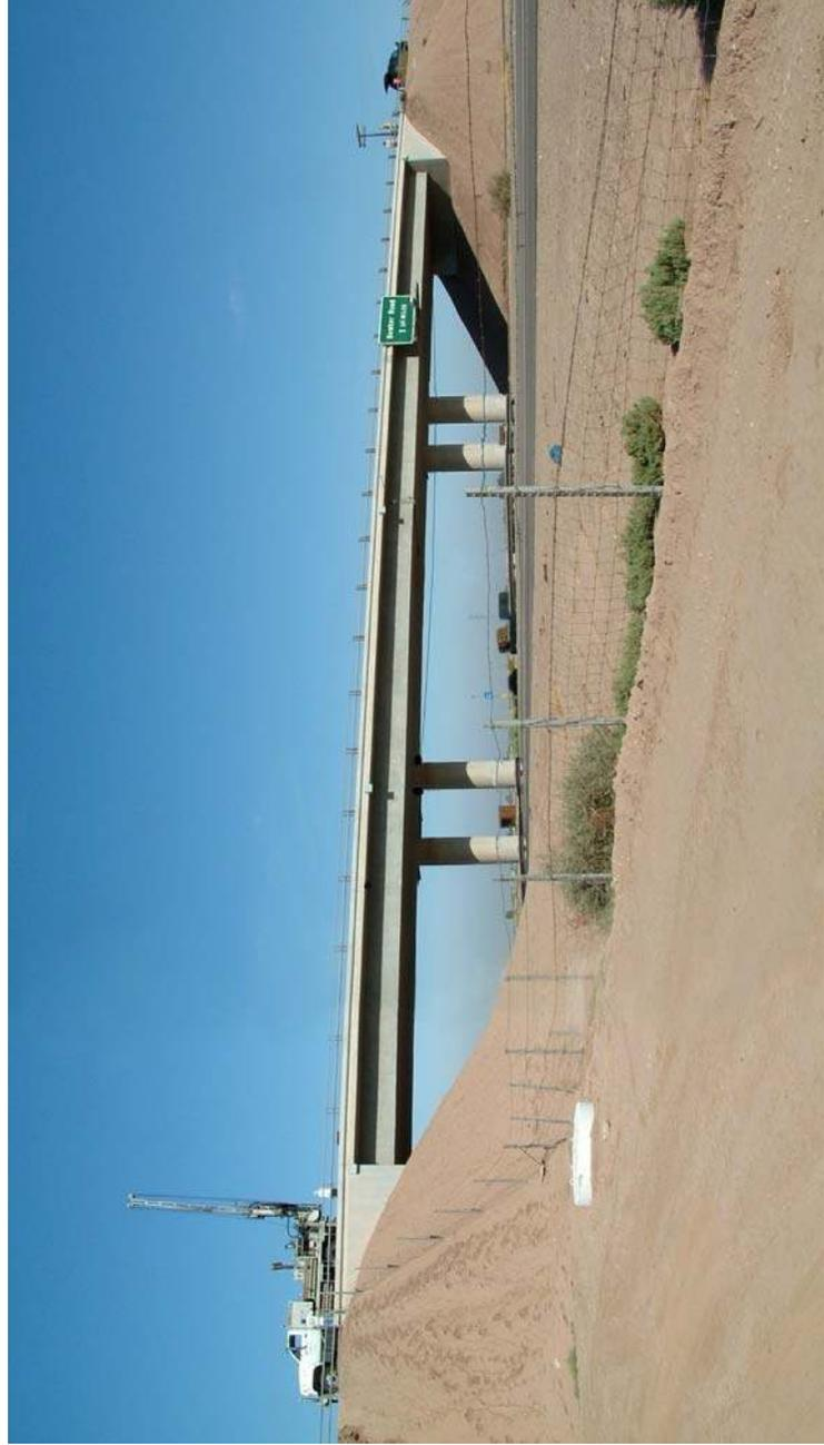
Figure 5.30: Tow-Columns Three-Spans Bent Bridge
