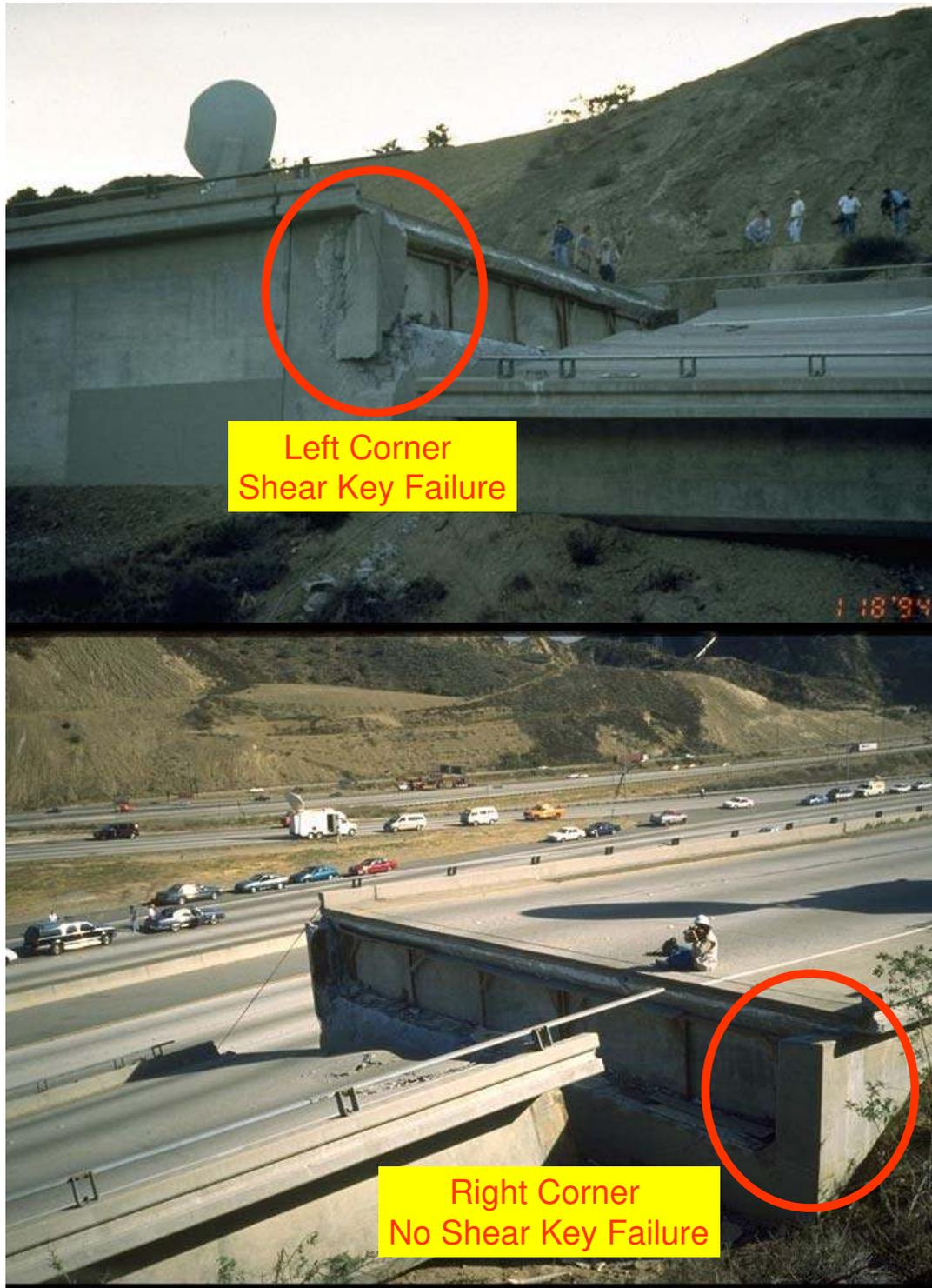
Figure 5.61: Shear Key Failure Due to Deck Rotation 1994 Northridge Earthquake
