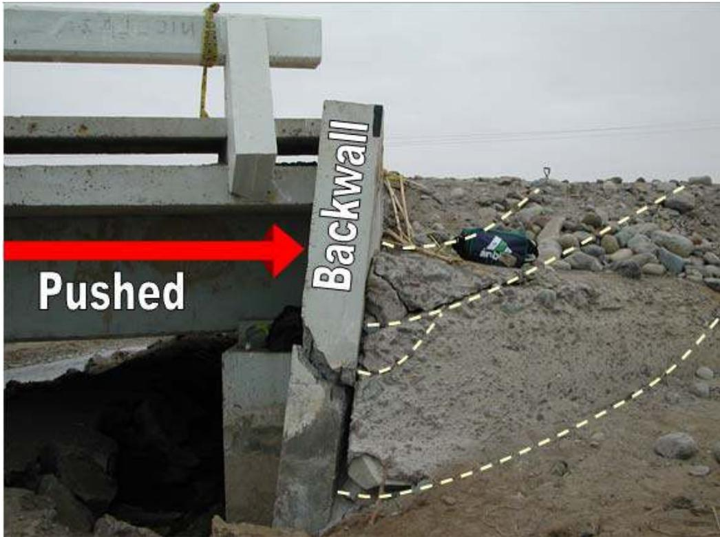
Figure 3.3: Example of Mobilized Passive Wedges
