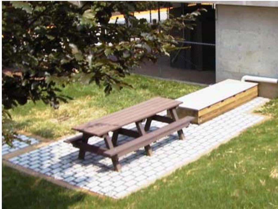
Figure 2.2 Infiltration Trench (Traver 2005)
