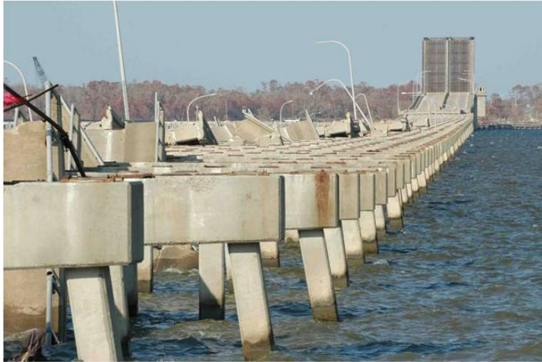
Figure 1.1: Damage to the U.S. 90 Biloxi Bay bridge caused by Hurricane Katrina. This photo is taken looking northeast from Biloxi 9/21/05 (source Douglass et al. (2006)).
