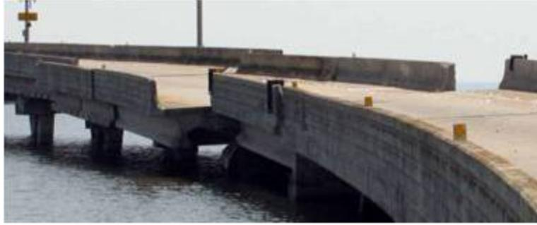
Figure 1.2: I-10 bridge, Mobile Bay, Alabama, damaged by Hurricane Katrina (source Douglass et al. (2006)).
