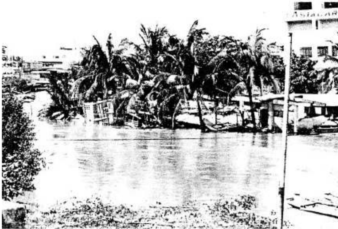
Figure 2-34: Lateral Spreading of Right Bank which pushed the wooden house into river (Wakamatsu et al, 1991)
