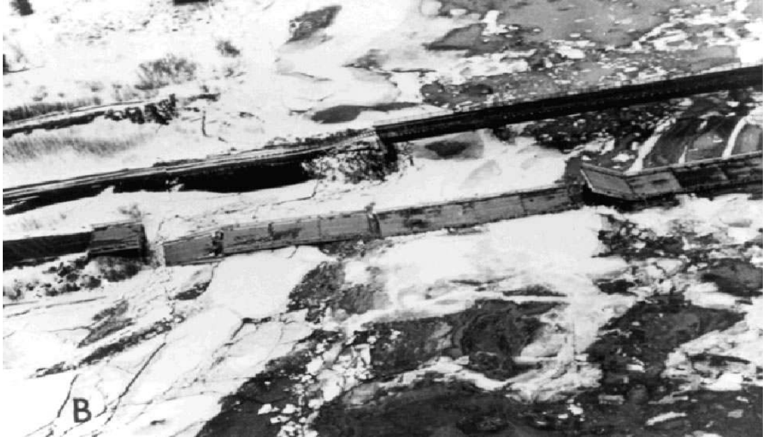
Figure 2-9: Damage to Railroad and Highway Bridge areas on Twenty Mile River (USGS5)
