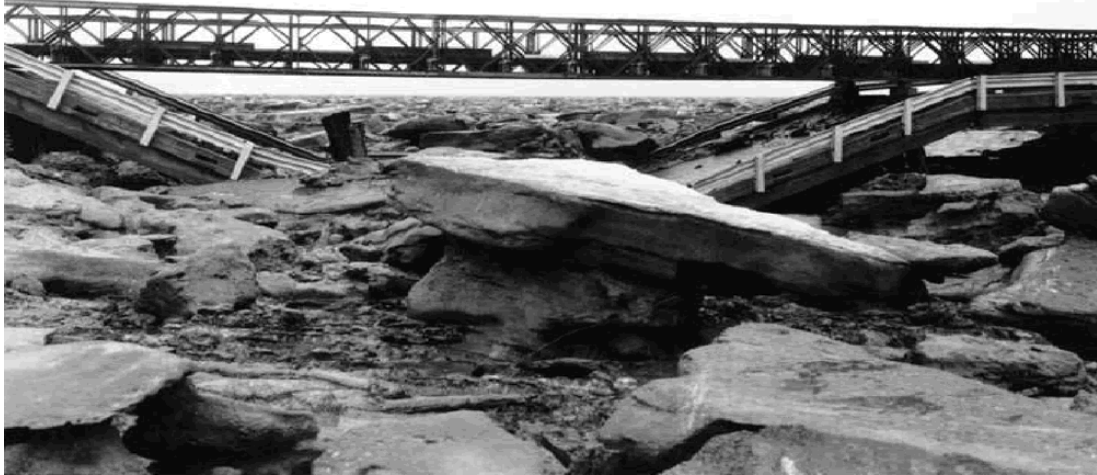
Figure 2-2: Damage to Twenty Mile River Bridge (Anchorage Museum of Arts and History, 1964)
