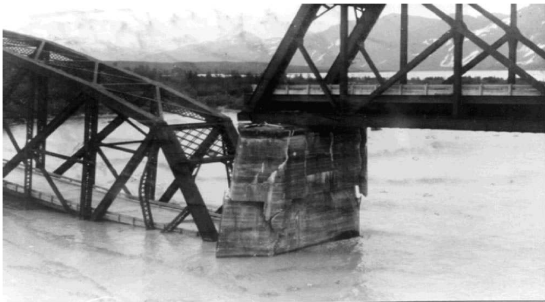
Figure 2-7: Span Collapse, Million Dollar Bridge, Copper River Highway (USGS4)
