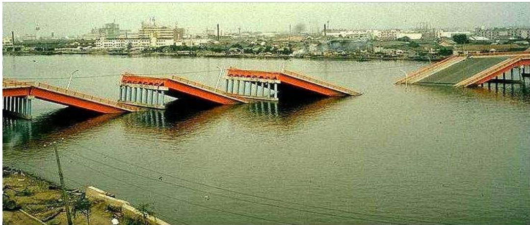
Figure 2-37: Showa Bridge Collapse (Kramer and Elgamal, 2001)
