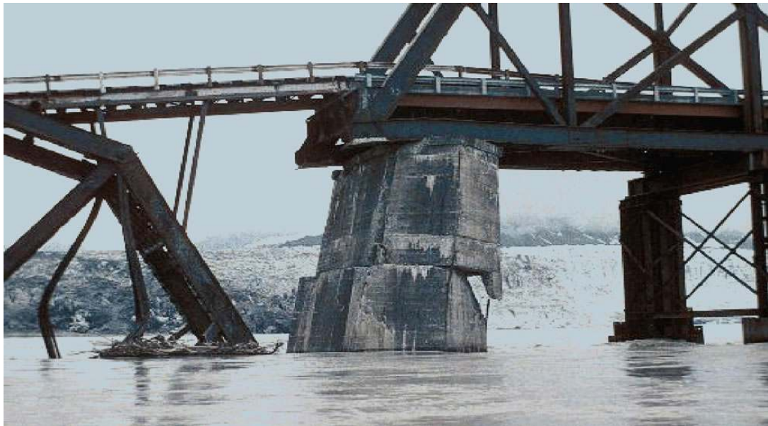
Figure 2-8: Temporary Bridging of Million Dollar Bridge, Copper River Highway (Molnia, B.)
