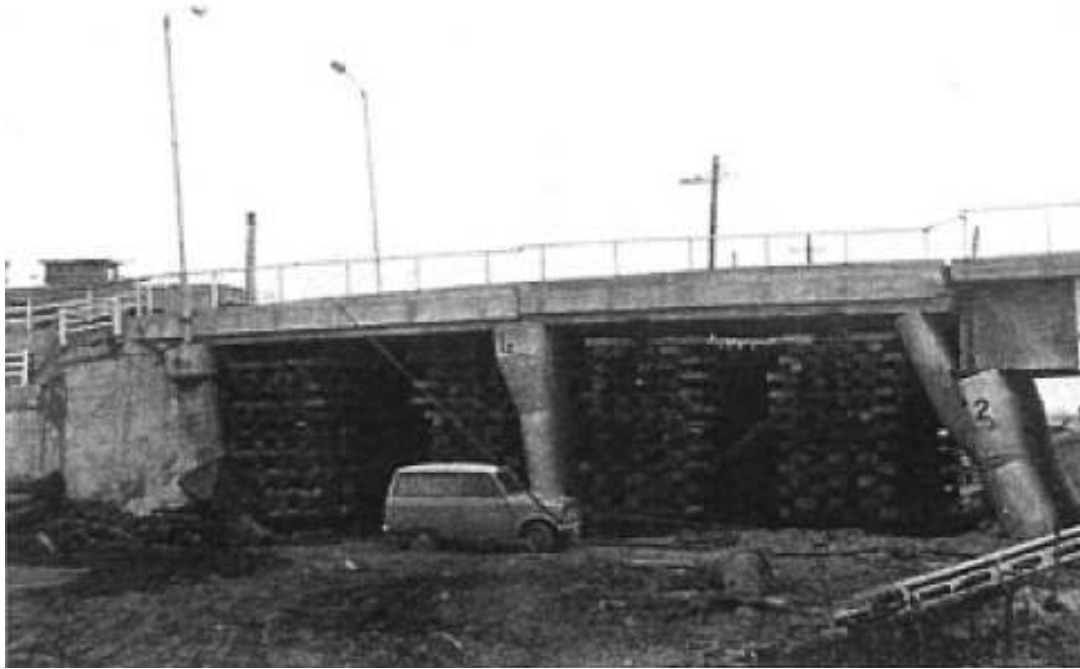
Figure 2-43: Damage to the Abutments and Piers of Yachiyo Bridge on the Left Bank (Hamada et. al, 1986)
