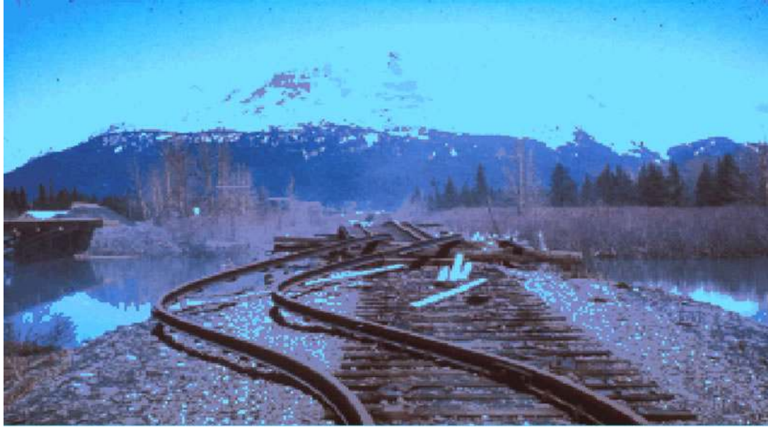
Figure 2-5: Railroad Approach Damage Due to River Bank Movement (USGS2)
