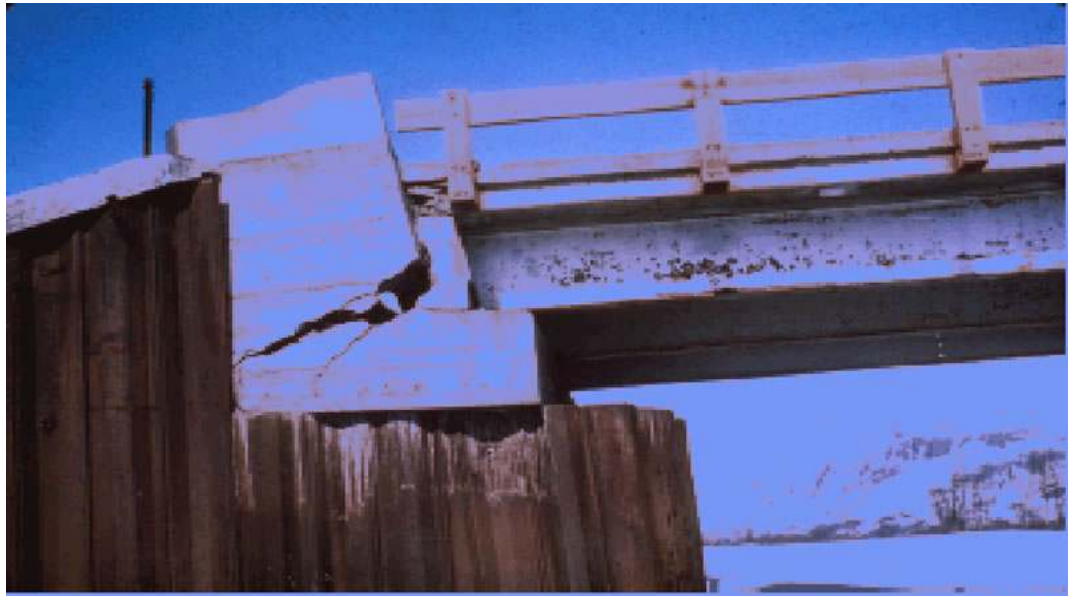
Figure 2-6: Railroad Approach Damage Due to River Bank Movement (USGS3)
